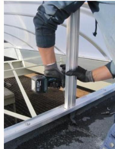
Fig 12 Fixation of end profile
