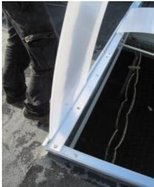
Fig 6 Gliding in the sheet into the lateral profile
