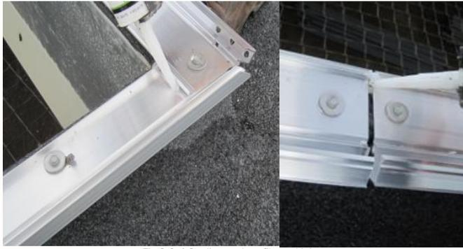
Fig 3 & 4 Sealing end profile and joints
