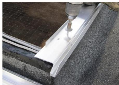
Fig 2 Installation of the end profile on the upstand
