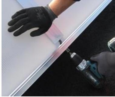
Fig 9 Fixation upper shells
