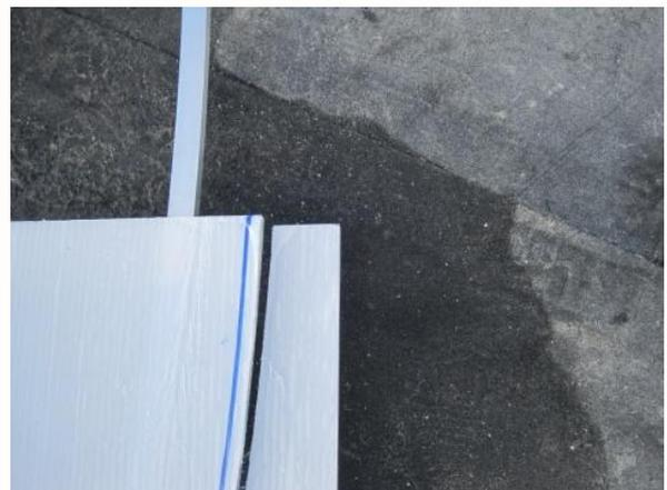
Fig 14 Cut off the end panel sheets at approximately 1,5 cm from the outside
