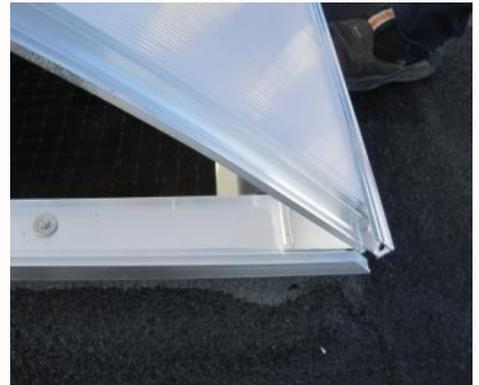
Fig 7 Mount the sheet on the other side too.
