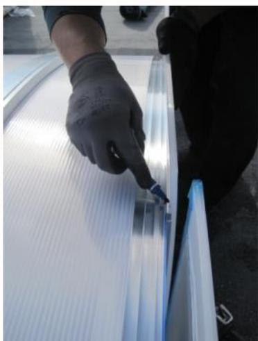
Fig 13 Mark off the form of the sheets
