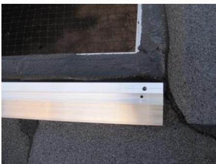
Fig 1 First lateral profile next to the upstand
