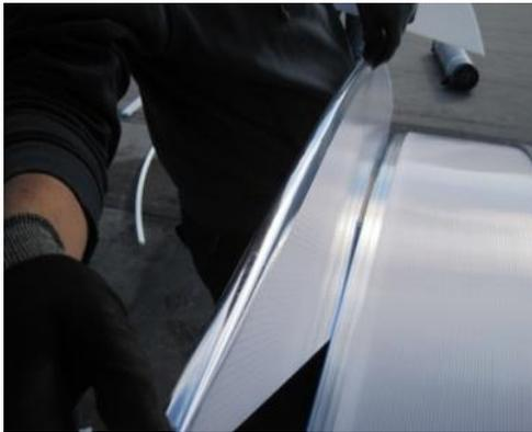
Fig 15 Tape off the sheet edges
