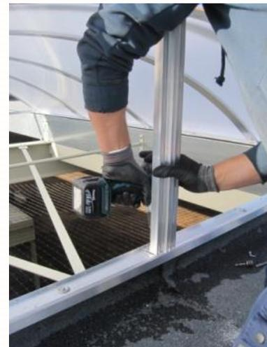
Fig 12 Fix end panel profile
