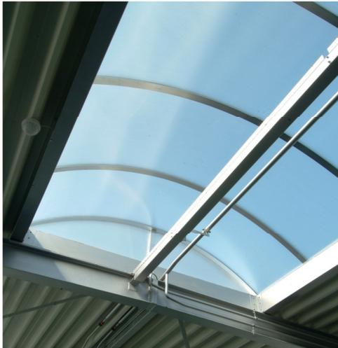
The glazing is bended between the upper scale and the supporting under scale. The bow profiles are only mounted at the ends on the horizontal longitudinal profile, which enables a quick installation and avoids differential tensions due to the dilatation of the plastic sheets. On request, rubber sealing can be used to diminish dilatation noise.
